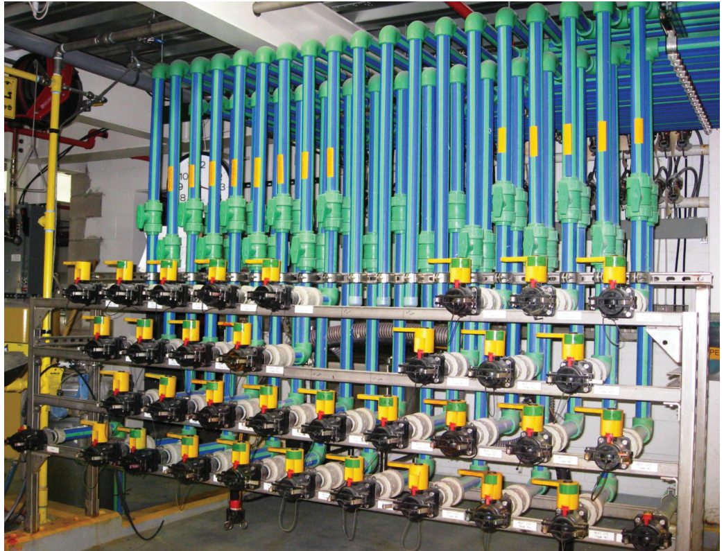
At a paper mill in Wisconsin, more than 19,000 ft of polypropylene pipe, connected by roughly 4,250 fittings and valves and more than 7,300 fusion welds, were installed with zero leaks at any of the joints.
