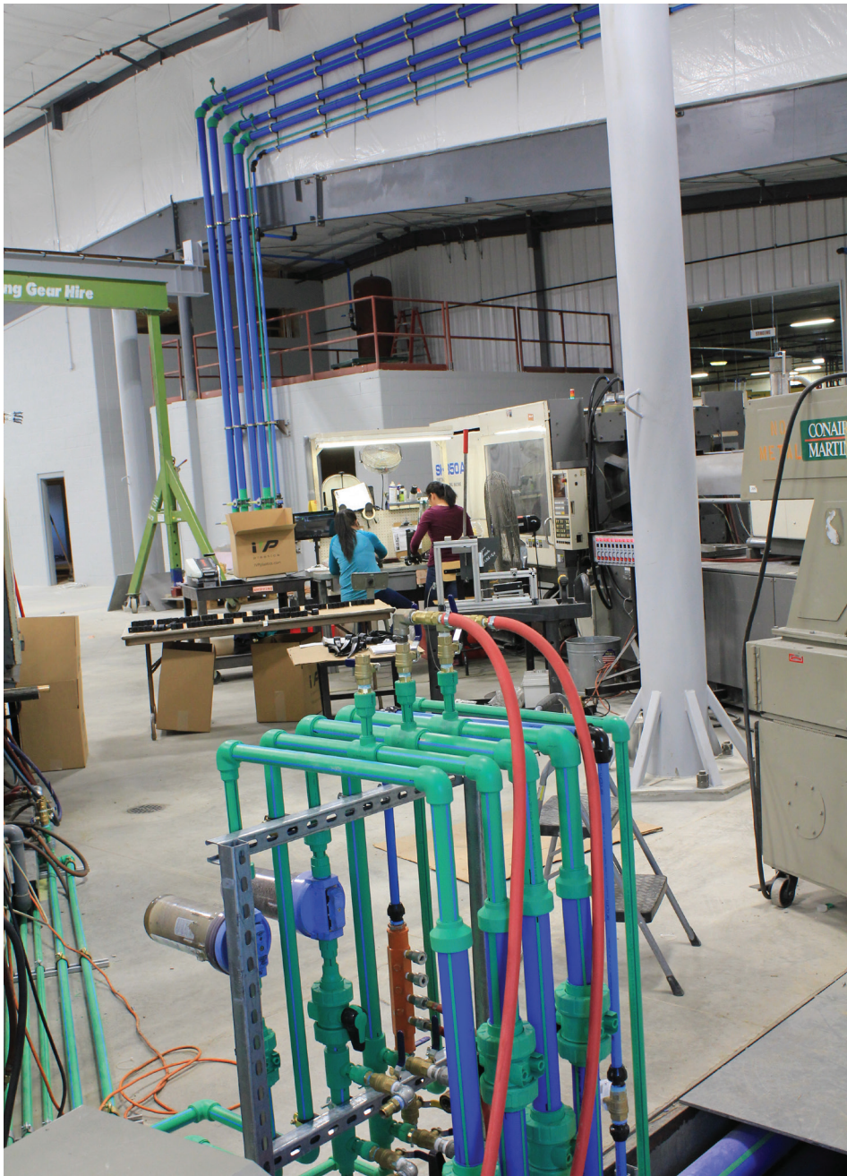
At a manufacturing plant in Illinois, polypropylene pipe in a trench provided the flexibility to accommodate frequent equipment re-configurations.
