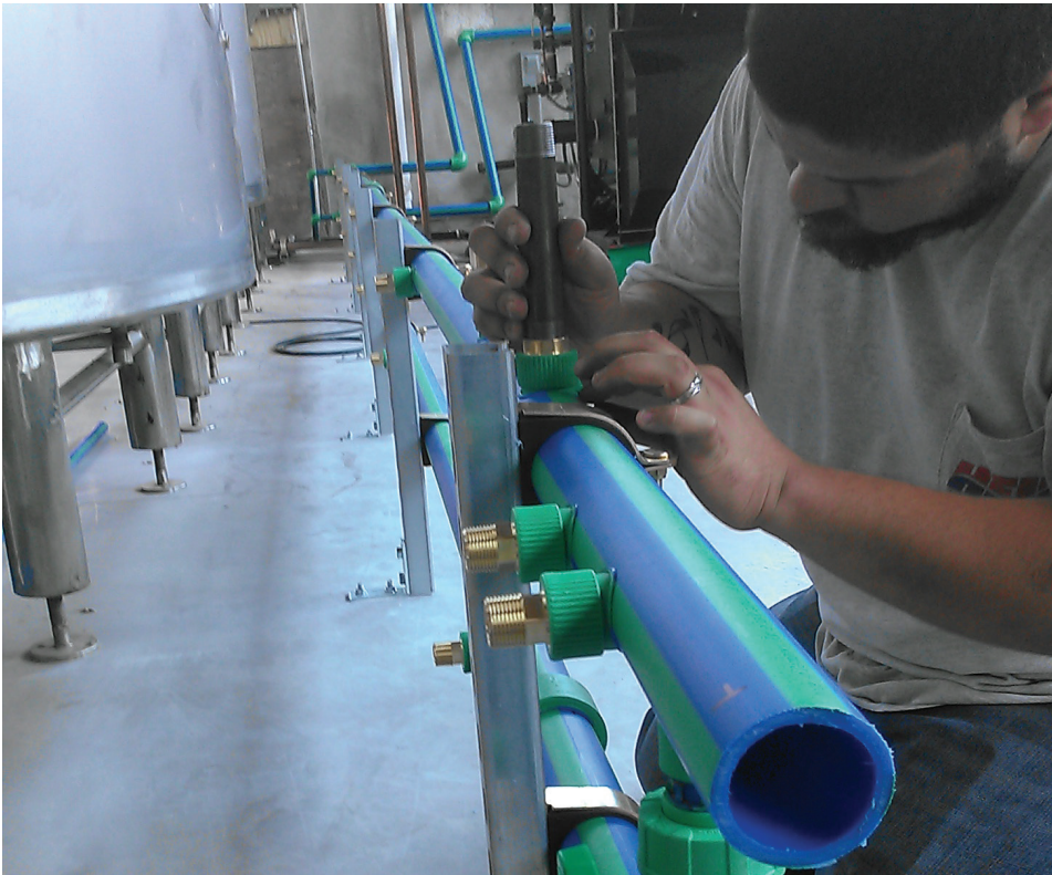
Lightweight, long-lasting, and easy to work with, polypropylene pipe typically represents a significant upgrade from metal pipe for craft brewers.
