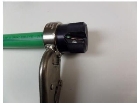
Cold Ring applied to the pipe at the base of the chamfer tool.
