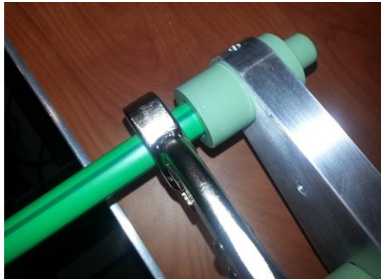
The heating tool is applied to the pipe until it hits the cold ring
