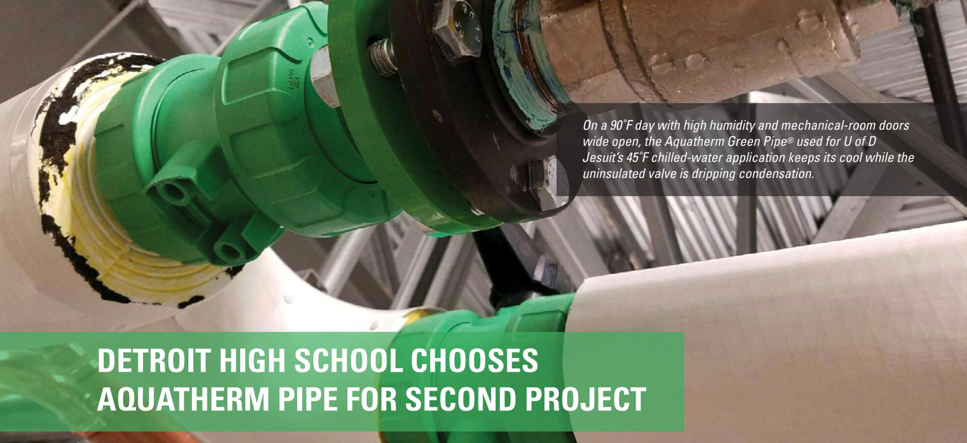
On a 90°F day with high humidity and mechanical-room doors wide open, the Aquatherm Green Pipe® used for U of D Jesuit's 45°F chilled-water application keeps its cool while the uninsulated valve is dripping condensation.
