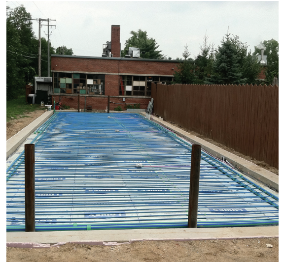
The ABC beer cave, which sits on top of this radiant grid, maintains a fairly constant temperature and never freezes – not even during the last couple extremely cold winters.
