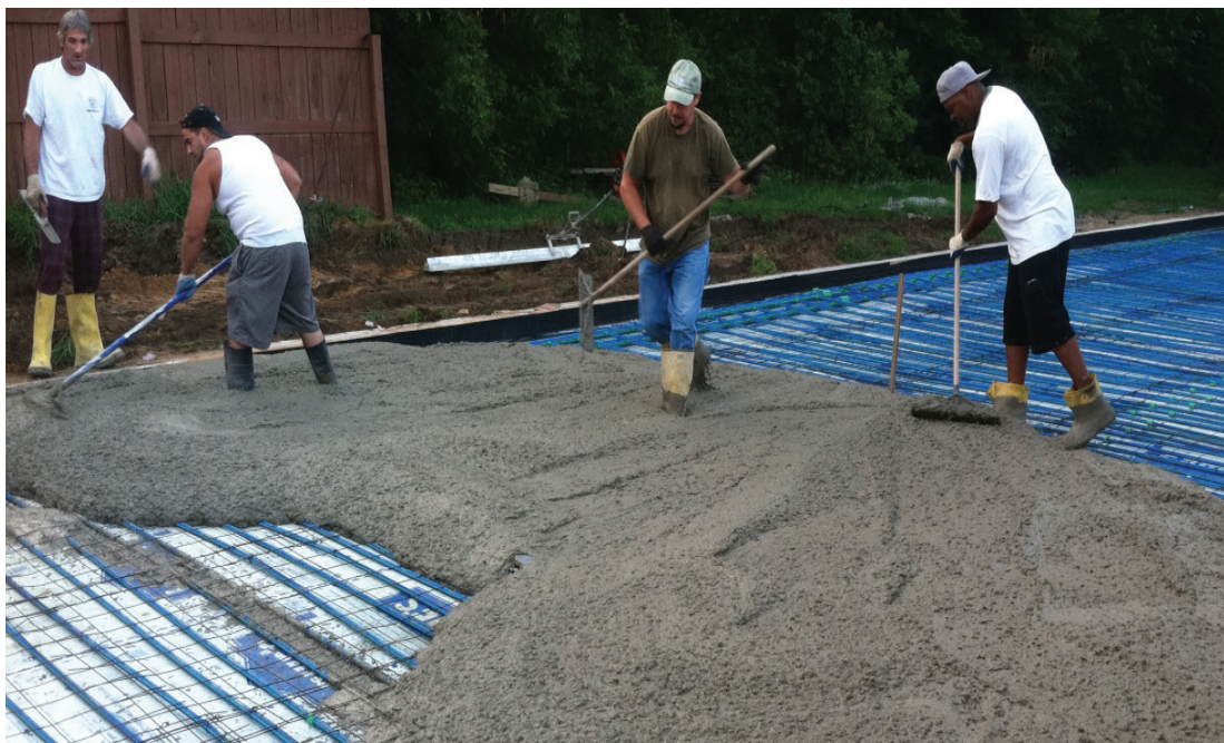
The ABC team installed 3,750 ft of ½-in. Aquatherm Blue Pipe which was embedded in the 6-in.-deep concrete floor of the beer cave (which is being laid in this photo).
