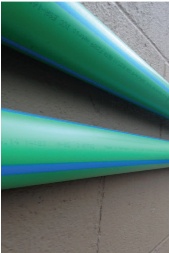
Two-in. Aquatherm Green Pipe® SDR 11 non-faser runs from the brewing vessels and tanks through a wall connection outside of the building, then runs underground to the packaging building that holds the beer until it's transferred into kegs, cans or bottles.
