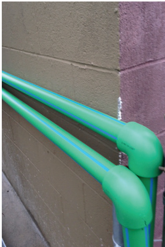
Two-in. Aquatherm Green Pipe® SDR 11 non-faser runs from the brewing vessels and tanks through a wall connection outside of the building, then runs underground to the packaging building that holds the beer until it's transferred into kegs, cans or bottles.
