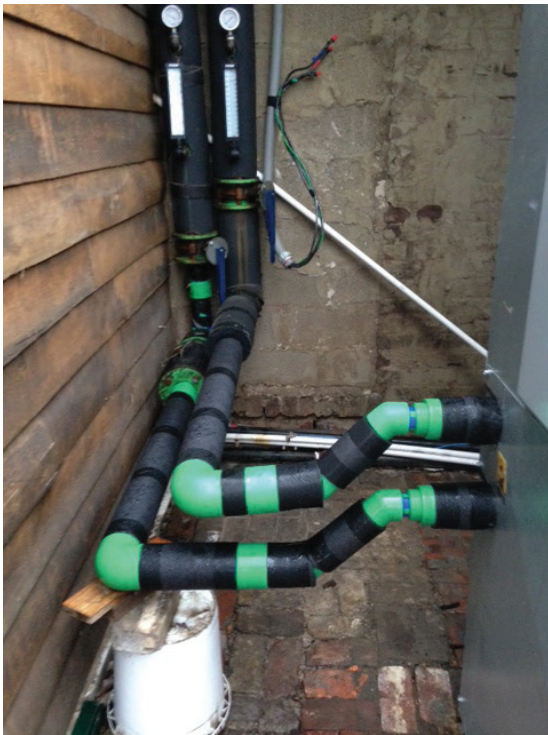
Having been impressed with the quality and performance of Aquatherm Blue Pipe on its chiller lines (shown here insulated and running from the chiller to the main brewery), Avondale's owners researched and ultimately selected Aquatherm Green Pipe for beer lines as well.
