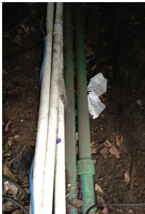
The 2-in. Aquatherm Green Pipe that carries beer from building to building was primarily buried 3 feet underground, but this section of pipe is in a crawlspace that goes from the main brewery and then underground to the packaging building.
