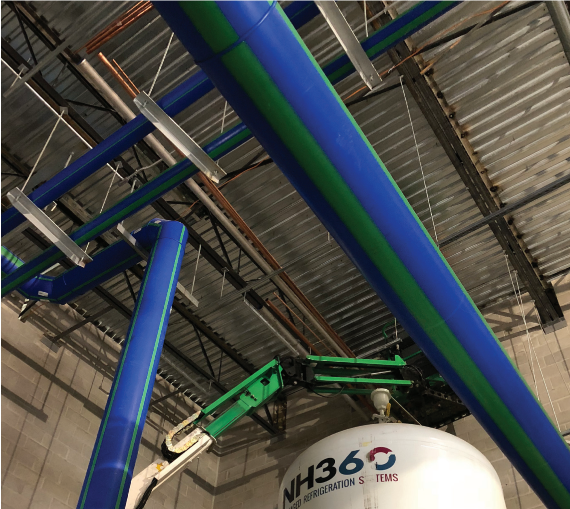
Offsite fabrication and the polypropylene-random pipe’s light weight allowed fabricated spools to be easily hung 25 to 30 ft above the floor.
