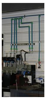
Aquatherm's unique heat-fusion welding technique provides joints that are more reliable than other methods. Heat fusion bonds both parts of a joint into a single, homogenous material without the use of chemicals or mechanical connections, which eliminates systematic weaknesses and fail-points in the pipe. The heat-fusion joints maintain the same properties as the pipe itself, so physical stresses will not damage their integrity. Fewer leaks mean lower maintenance costs.
