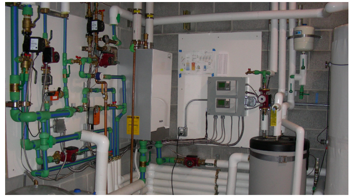
The mechanical space at Carl Pond's contracting business was left open intentionally in a corner of the warehouse to show off the company's green technology offerings and skills. Aquatherm Climatherm was used to connect the various valves, pumps, TEC controllers, and the condensing boiler, in addition to the other components.
