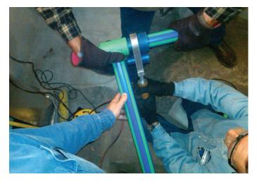
The Climatherm product was approved for Ohio commercial code hydronic use and was approved for the residential application with the local building department. "Blue Pipe holds dimension with temperature changes. It was temperatureand pressure-rated for the application and was easily joined using the socket fusion method. We're very familiar with that method through our work with fusion welding high density polyethylene pipe (HDPE) as geothermal system contractors," Persons explained.
