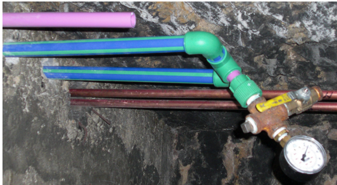
Using Aquatherm’s heat fusion to connect the pipes in this tight crawl space was considerably easier and safer than using a welding torch, according to the Monroe staff.
