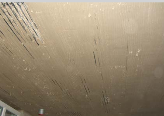
Ceiling heating plaster ceiling
