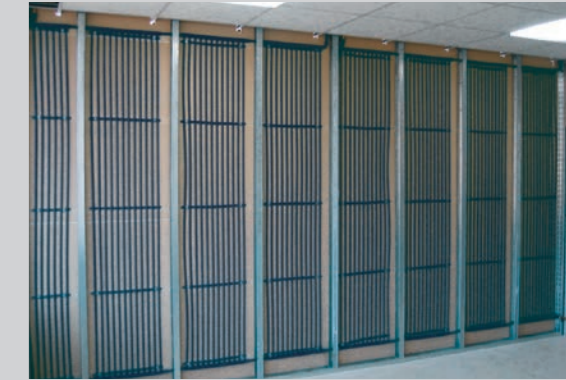
Drywall with plasterboard ceiling
