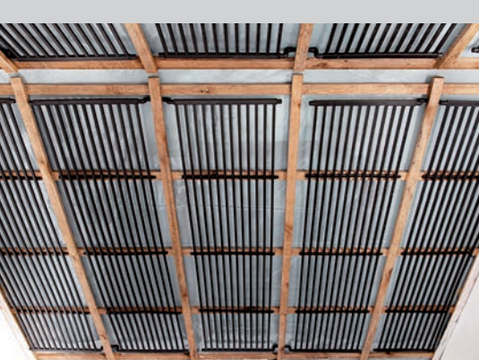
Plasterboard ceiling with wooden base
