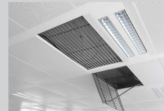
Metal tile ceiling
