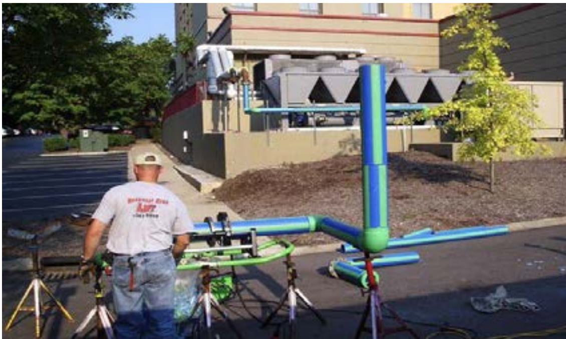
Jamie Hassett worked as a service manager for another company in 2008 when he was butt fusing 6-in. Aquatherm Blue Pipe® for this chiller piping retrofit at the Embassy Suites Nashville Airport. He went on to form his own company, Demand Mechanical, a few years ago and used Aquatherm Green Pipe® on another retrofit at the hotel
