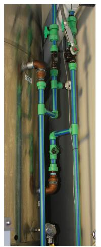
and Air Conditioning, the brewery's mechanical contractor. "At the time copper was very expensive and from a brewer's perspective, Aquatherm gives you a hydrostatic, pneumatic pipe with a pressure test of 200 psi," Crompton said.
