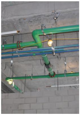
approximately 3,000 linear feet of Climatherm piping, including roughly 855 feet of 2-inch, 330 feet of 1 ½-inch, 470 feet of 1 ¼-inch, 920 feet of 1-inch and 420 feet of ¾-inch.
