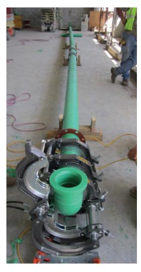
be extremely cost effective. One of the unique construction aspects of the project emerged from the value engineering of the mechanical and plumbing systems after the local plumbing and HVAC distributor recommended polypropylene-random piping for the domestic hot and cold water and chilled water for the stadium.
