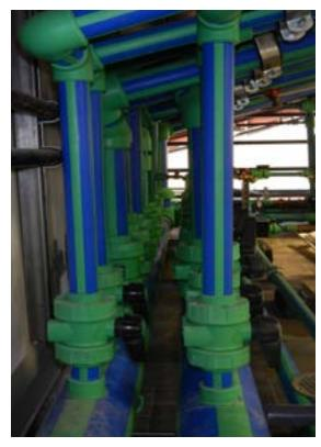
Van Dort used both socket and butt fusion to assemble the complex network of piping. The contractor used McElroy Spider™ equipment for fusion installations of Aquatherm pipe and fittings that were 2-inches and larger. This device features a worm gear drive with parallel link system to bring pipe and fittings together evenly and under control. For smaller pipe sizes, Van Dort used socket fittings and hand-held welding irons to join pieces of pipe together.
