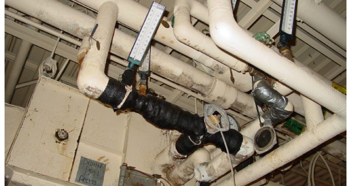
The existing HVAC system was ready for an overhaul and some of the existing pipes were too.
