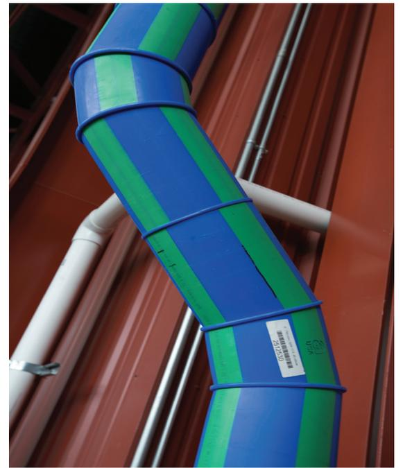
The team at Founders takes a lot of pride in keeping their brewery clean. “This was the cleanest brewery we’ve ever set foot in,” Strouse explained. “That is what led us to install Aquatherm piping in this facility. It’s wash-down rated and leak free after you install it.” Strouse added that using Aquatherm over copper provided some material savings, though specific figures weren’t available.
