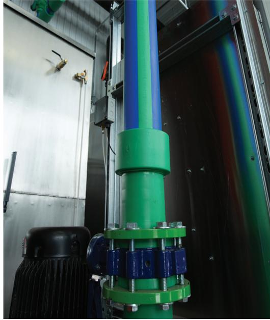
Anes provided training on the Aquatherm piping and the team used Aquatherm welding equipment rented from Columbia Pipe & Supply Co. to install the piping.
