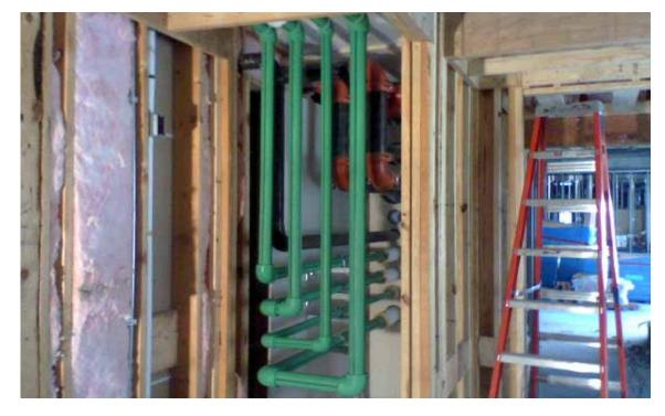
we need to do." Beginning in October 2011 Midstate began installing more than 23,000 ft of Aquatherm Green Pipe ranging in size from ½-in. to 4-in. for domestic water supply in three buildings.
