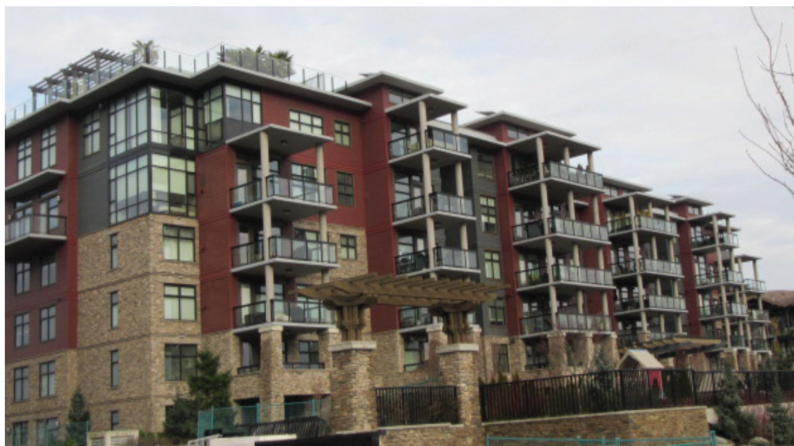
GML's 77th Aquatherm project is under way at Tsawwassen Springs phase 4, a 4-story, 63-unit residential building in Tsawwassen, BC. GML Mechanical is using Aquatherm pipe for the domestic water piping in the mechanical room and all the mains. Aquatherm PP-R piping also was used on phases 1, 2, and 3 of the project.
