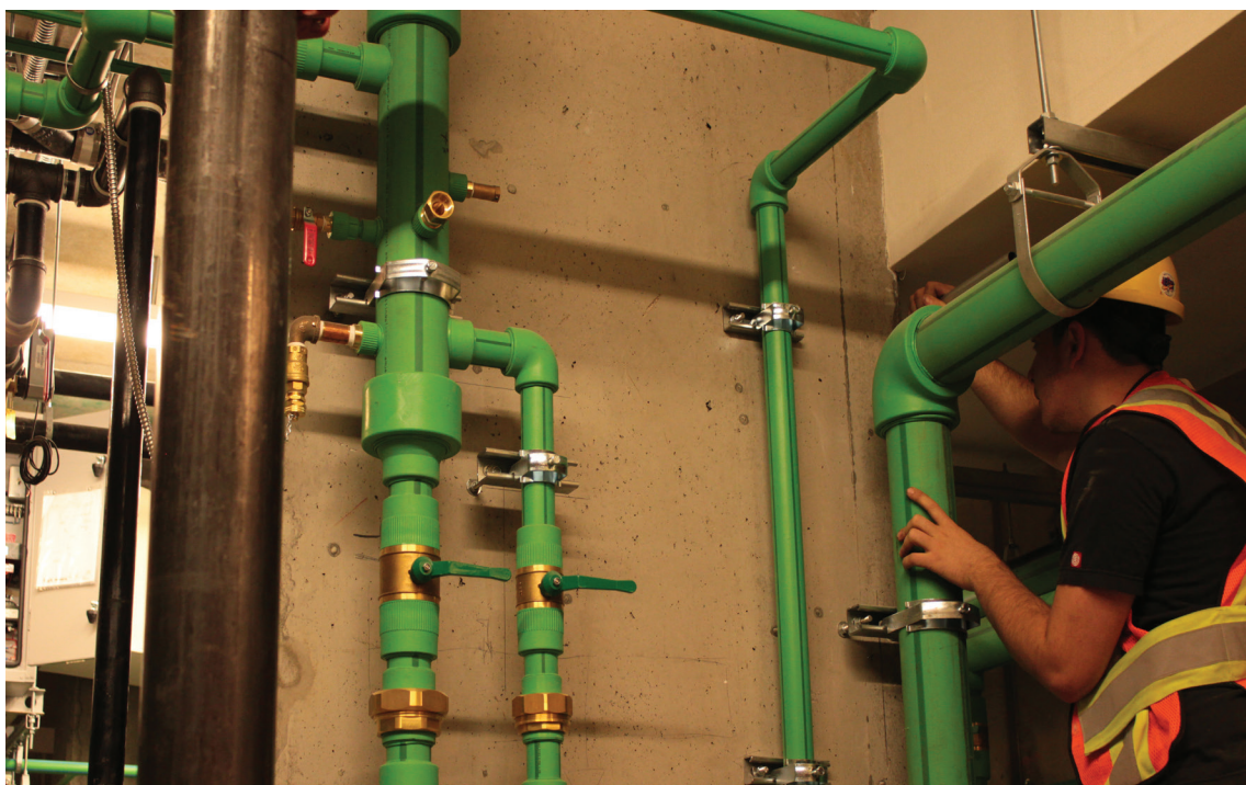
GML has installed Aquatherm on several high-rise projects including this one, which was built in the Vancouver area in 2012. The company’s estimators appreciate that it’s much less expensive than copper pipe and doesn’t fluctuate in price the way commodities such as copper do.
