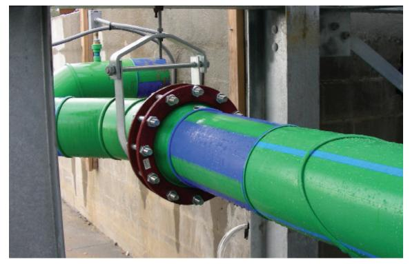
One of the first challenges to Phase 1 was choosing and installing a new piping system. During Hurricane Katrina, Bay St. Louis experienced a storm tide more than 30-ft deep, causing damage to the framework of most local buildings; the medical center's existing domestic water and chilled and heating water steel and copper piping systems needed to be replaced.
