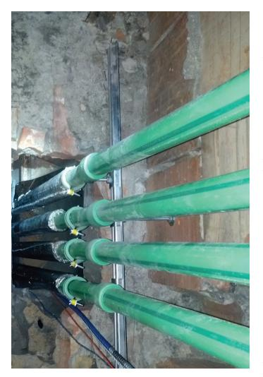
After a half-day training conducted by NextGen and renting the proper fusion welding irons, the team used approximately 200 ft of ½-in. to 2-in. Aquatherm Green Pipe® to run from the mechanical room to the new fcus on the second floor and provide heating and cooling to the office spaces. The installation proceeded remarkably smoothly considering it was the first Aquatherm installation for HMS and Pinnacle.
