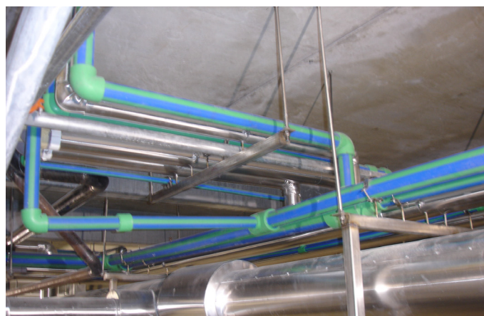
While stainless steel was used some areas of the plant due to aesthetics, over 4,000 lineal feet of Aquatherm was used for compressed air, cow water, and door and foot foamers.
