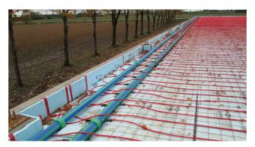
Since — at the request of Raftis — the hydronic installation needed to be installed on one heating zone, the design team specified a very efficient Aquatherm Pipe reverse return header system — whereby supply and return lines are embedded in the concrete and run from the boiler room to supply water to the floor heating circuits.
