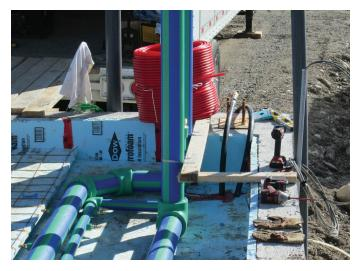
The building is 265 ft  $\times$  150 ft; therefore, the header was divided into three sizes 1) to reduce material costs and 2) because larger pipe diameters would not be needed to supply the flow rates required to the circuits at the end of the building. The three sizes of Blue Pipe also meant the installation did not necessitate many different sizes of fusion heads.
