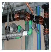
He added that his crew typically realized labor savings of 20-25% versus copper since there is no cleaning and fluxing of the pipe, and due to its light weight relative to metal. TJ Dyer installer Dexter Campbell – a 30-year industry veteran – added that while there is a learning curve involved with the Aquatherm
