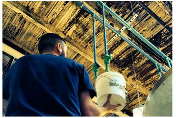
total of approximately 400 ft of Aquatherm Green Pipe<sup>®</sup> and Aquatherm Blue Pipe<sup>®</sup> ranging in size from ½-in. to 1½-in.
