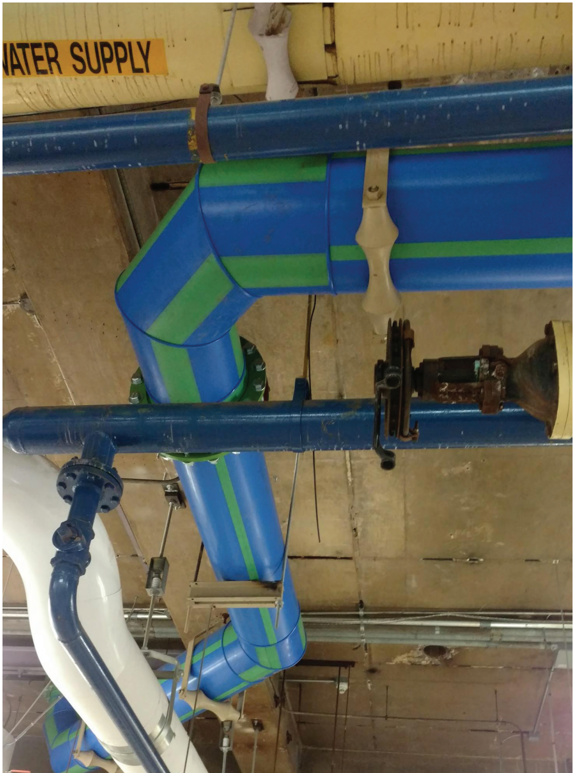
The easy configurability of Aquatherm Blue Pipe allowed it to work well in “heavy traffic” at this project.
