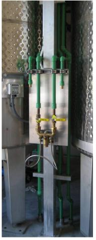
concerns that come with metals, including corrosion and electrolysis. "The entire Napa valley is full of silica. If you use regular water treatment, it would glaze the inside of the pipe walls," said Costa.
