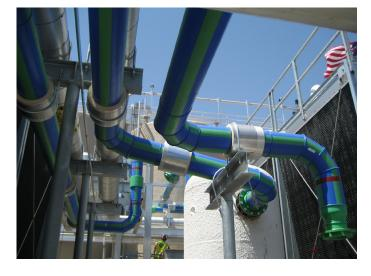
air. In fact, Aquatherm piping can be used for general utility services such as cooling water, reverse osmosis/deionized water, compressed air, inert gases, glycol and others.
