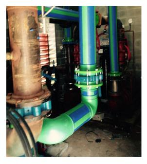
"If we had used steel on this project, we would have had to have rigging equipment onsite and put every joint together by hand. In addition, all outlets would have had to be welded, which is a huge fire hazard," he said.
