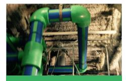
"If we had used steel on this project, we would have had to have rigging equipment onsite and put every joint together by hand. All outlets would have had to be welded, which is a fire hazard."
