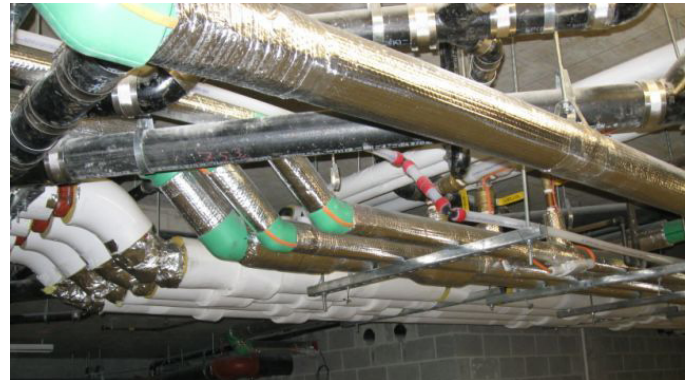
While PP-R has a natural R-value of 1, Aquatherm Advanced, a foil wrap, was added to meet flame spread code requirements.
