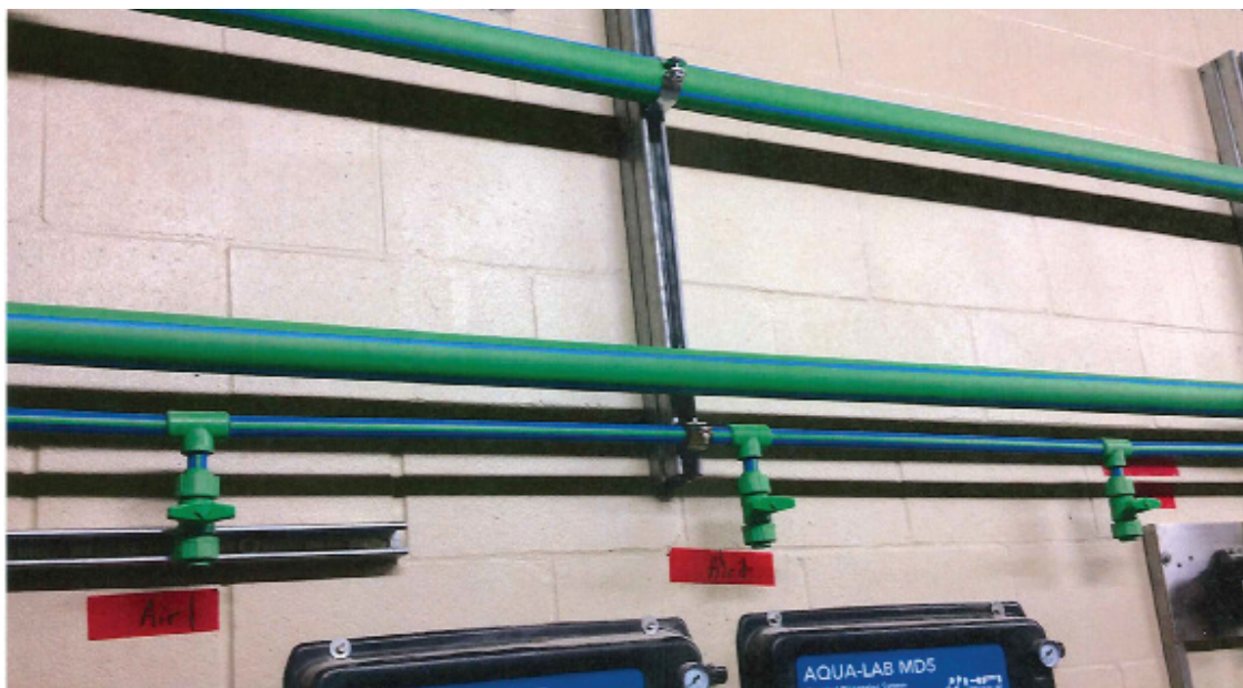
The various colors of Aquatherm pipe reflect the different applications for which the products are designed. Here, the Blue Pipe is carrying compressed air while the Green Pipe carries reverse-osmosis water.
