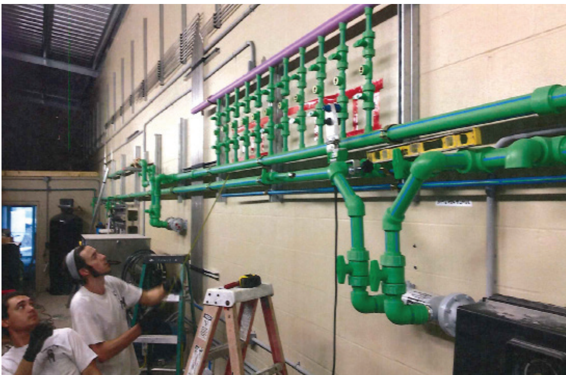
Closest to the ceiling, roughly 100 ft of 2-in. Aquatherm Lilac Pipe® channels reclaimed water for the car wash’s initial cold-water rinse and scrubbing stages.
