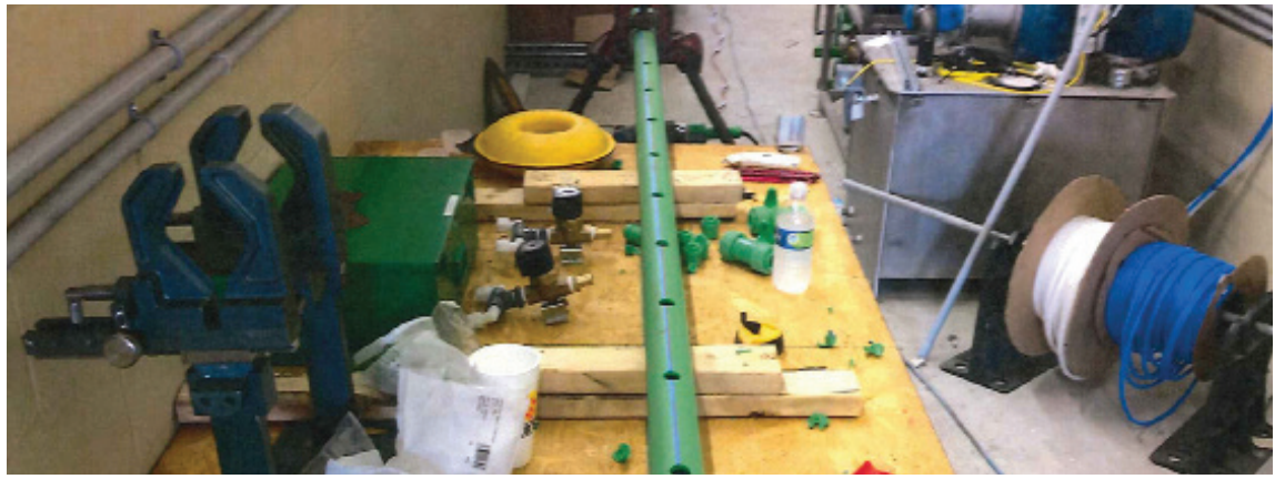
Prefabrication of Aquatherm pipe often leads to significant labor savings on the jobsite. On bigger jobs, it can also make sense to use the company’s Custom Prefabrication Services.
