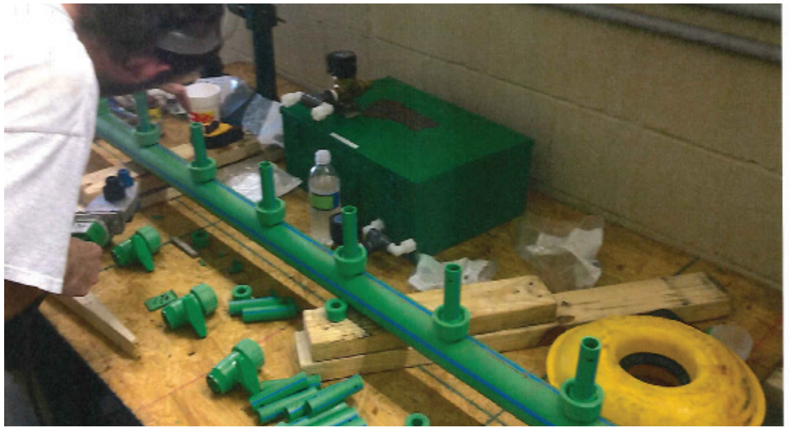
Despite working with Aquatherm for the first time on this job, the installers at Leon’s Plumbing found it “fun to install” and were “excited to go to work.”
