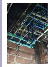
Heat fusion bonds both sides of a joint into a single, homogenous material without the use of chemicals or mechanical connections, which eliminates systematic weaknesses and fail-points in the pipe. The seamless heat fusion connections do not require an open flame or burn permit like soldering does (the heating iron, which reaches 500°F, is plugged into a standard 110V outlet).
