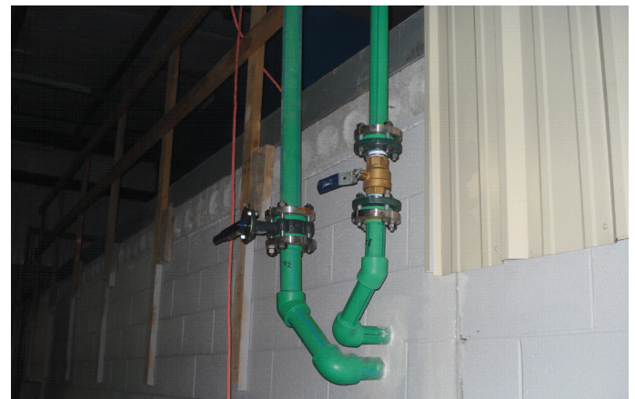
Aquatherm Greenpipe provided a superb alternative to copper at a time when the metal was extremely costly.
