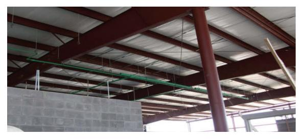
reduces concerns about the cost (and theft) of copper and is designed specifically for potable water applications.
