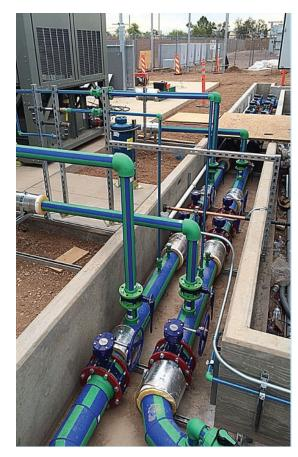
form connections; heat fusion bonds both sides of a joint into a single, homogenous material without the use of chemicals, adhesives or mechanical connections, which eliminates systematic weaknesses and potential failpoints in the pipe. The seamless heat-fusion connections, combined with the piping's resistance to corrosion and abrasion, help to ease leakage concerns.
