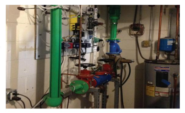
to commit to future costly repairs. Instead of digging up the concrete floor—another pricey solution—Mitchell hung 300 ft of 3-in. Green Pipe with MF from the ceiling in Walraven hangers for a domestic cold water line, 100 ft of which was suspended over an Olympic-sized swimming pool.
