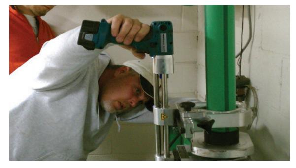
seamless heat-fusion connections, combined with the piping's resistance to corrosion and abrasion, help to ease leakage concerns.
