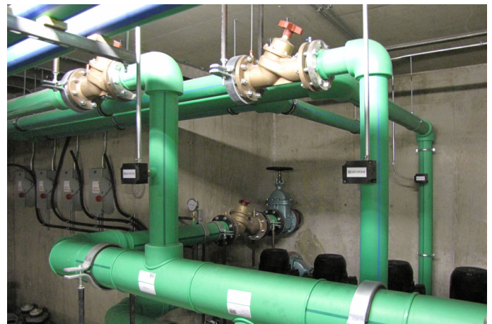
While Sandhill Mechanical was new to heat fusion butt welding of the 6-inch and 8-inch pipe the crew became experts at it quickly.
