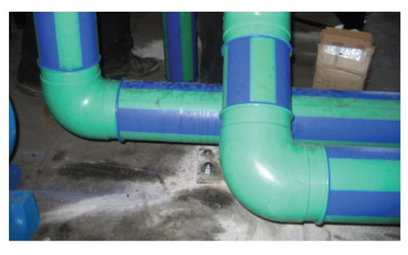
typically carried 40-50 °F water from the plant's four chillers at 40-60 psi to the different process areas.
