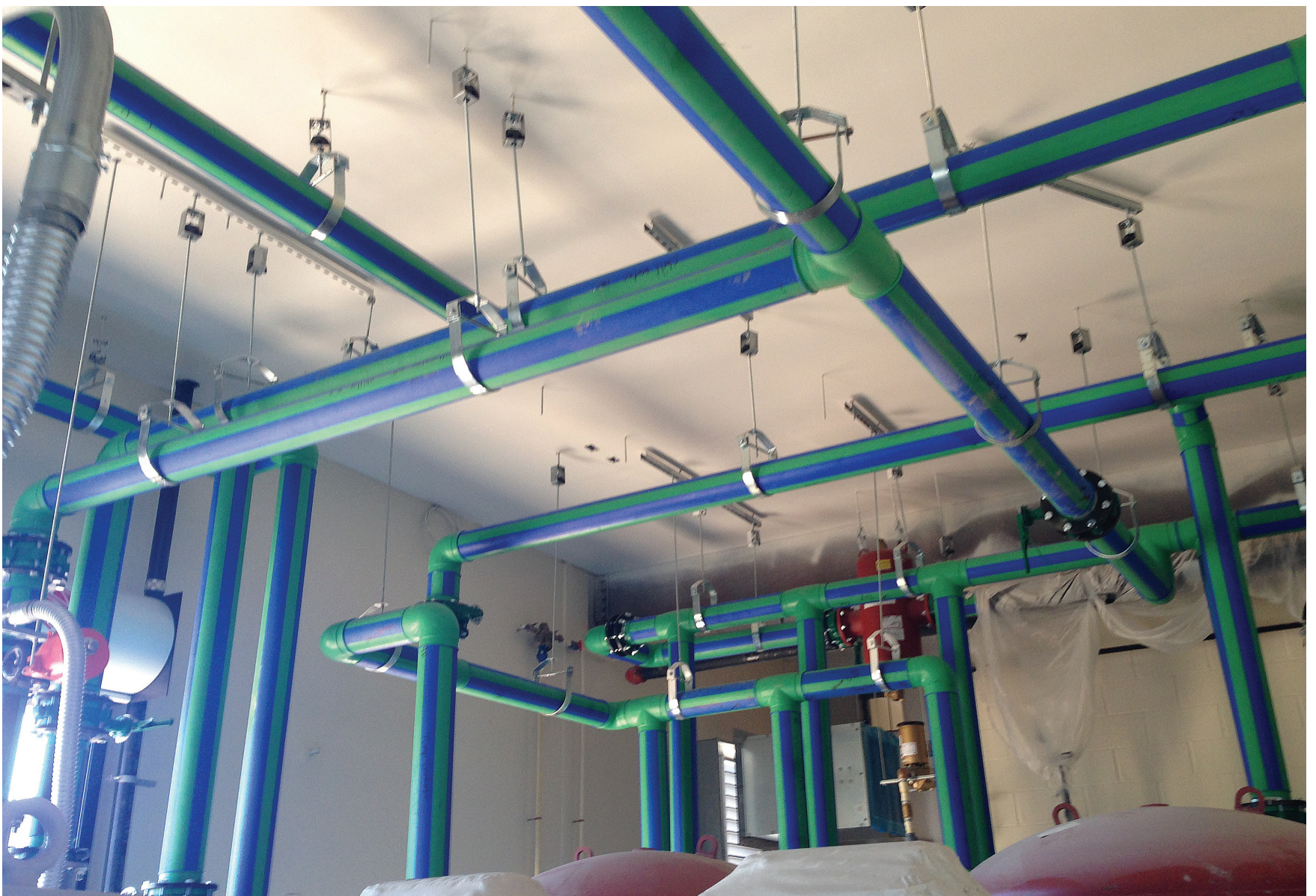
Blue Pipe with MF technology is extruded with a middle glass fiber layer that reduces expansion by 75% compared with other
