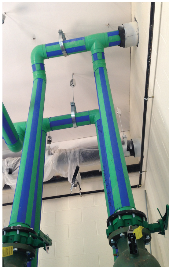
Blue Pipe with MF technology is extruded with a middle glass fiber layer that reduces expansion by 75% compared with other
