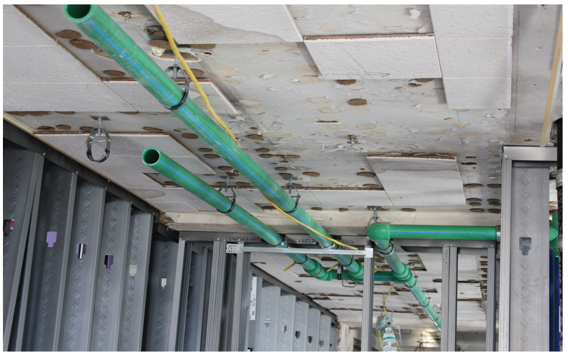
More than 8,300 ft of Aquatherm piping, ranging from 3/4-in to 12-in, helped make this project a success.
