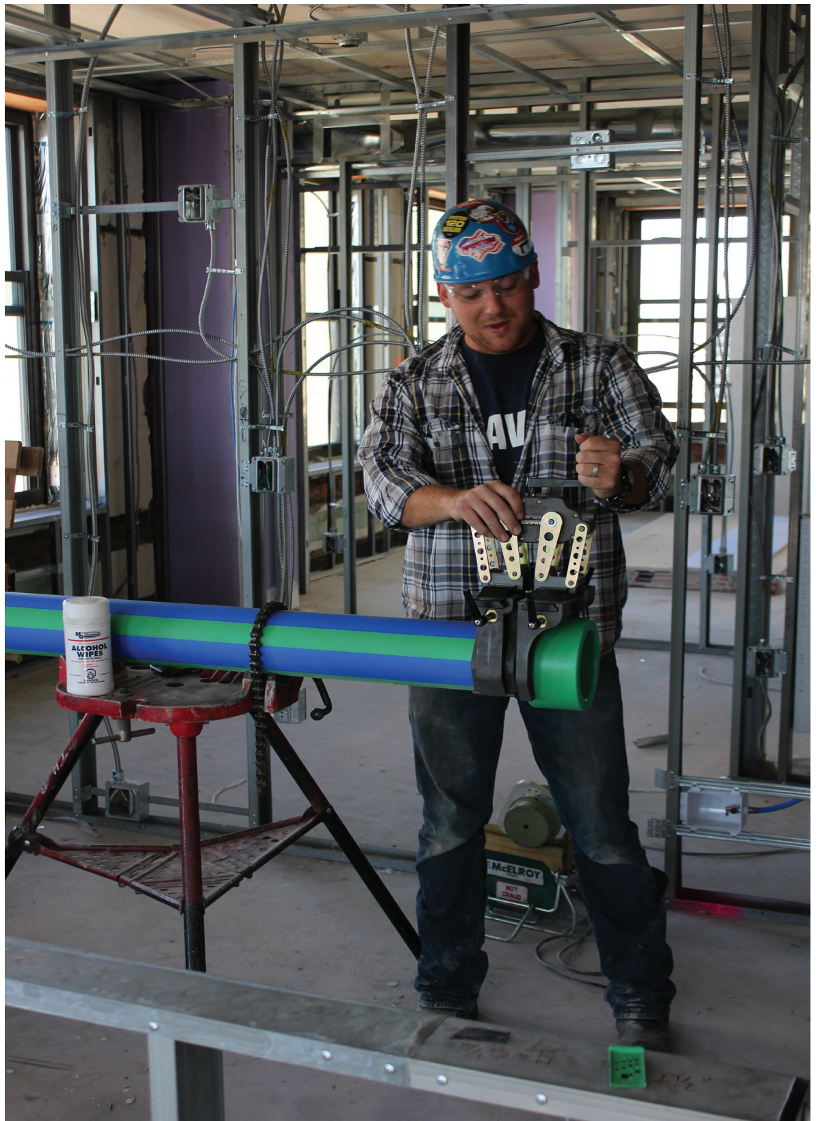
The project’s tradesmen appreciated Aquatherm pipe because it is lighter and cleaner to work with than steel pipe.
