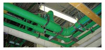
Since Aquatherm is corrosion- and rust-proof, those issues were automatically removed from the list of concerns. Additionally, Strunk explained that he was also impressed with the ability to easily tie-in to the pipe and do repairs using Aquatherm's fusion outlets. The fusion outlets are huge labor savers since they allow installers to simply drill into the supply pipe, then heat fuse the fusion outlet fitting into place wherever needed.
