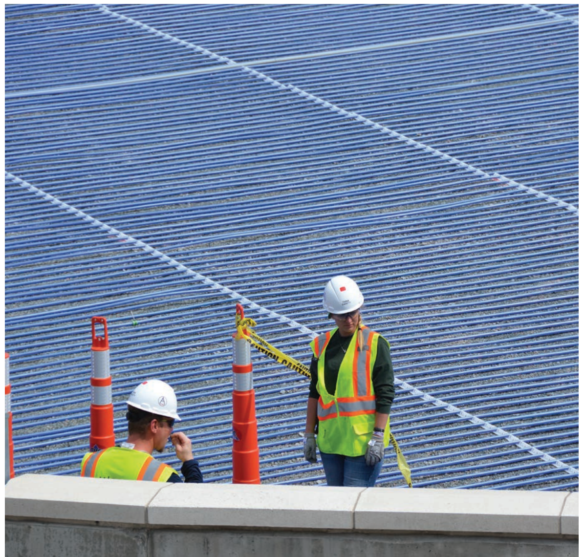
Two installers in front of a sea of blue coils installed on the TCF Bank Stadium field before the coils were covered with sand.
