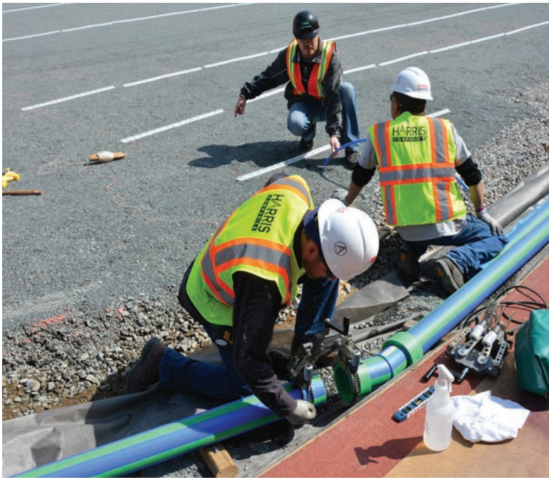
Installers connecting manifolds using the McElroy Spider™ 125 .
