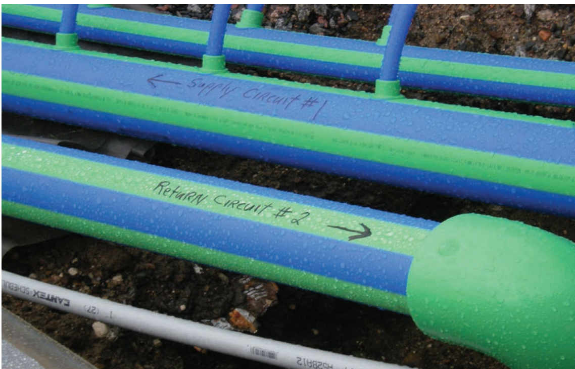
Close up of the supply and return lines, which carry DOWFROST™ HD Inhibited Propylene Glycol-based Heat Transfer Fluid (this photo was taken on a rainy day, thus the water droplets on the piping).
