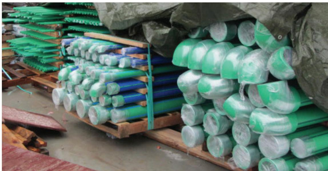
*Spools fabricated by Aquatherm's Design and Fabrication Services await installation at UBC Gage South. 10 pallets of fabbed Green Pipe® and Blue Pipe® were delivered to the site.*
