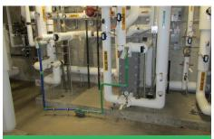
"The light weight [of Aquatherm pipe] has been a real bonus. With copper, we could only put 12 ft in the air at a time. Here we can fuse together 20- or 30-ft runs, and put the whole length up in the air without worrying about the weight."
