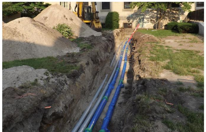
throughout the pipe-laying portion of the project. While the team had budgeted for the trench to be uncovered (and an excavator operator required onsite at his hourly rate) for eight or nine days, it only took six days. "If we had put steel or welded pipe in, it would have taken a lot longer. It went fast, faster than we were expecting," Bobrowski added.
