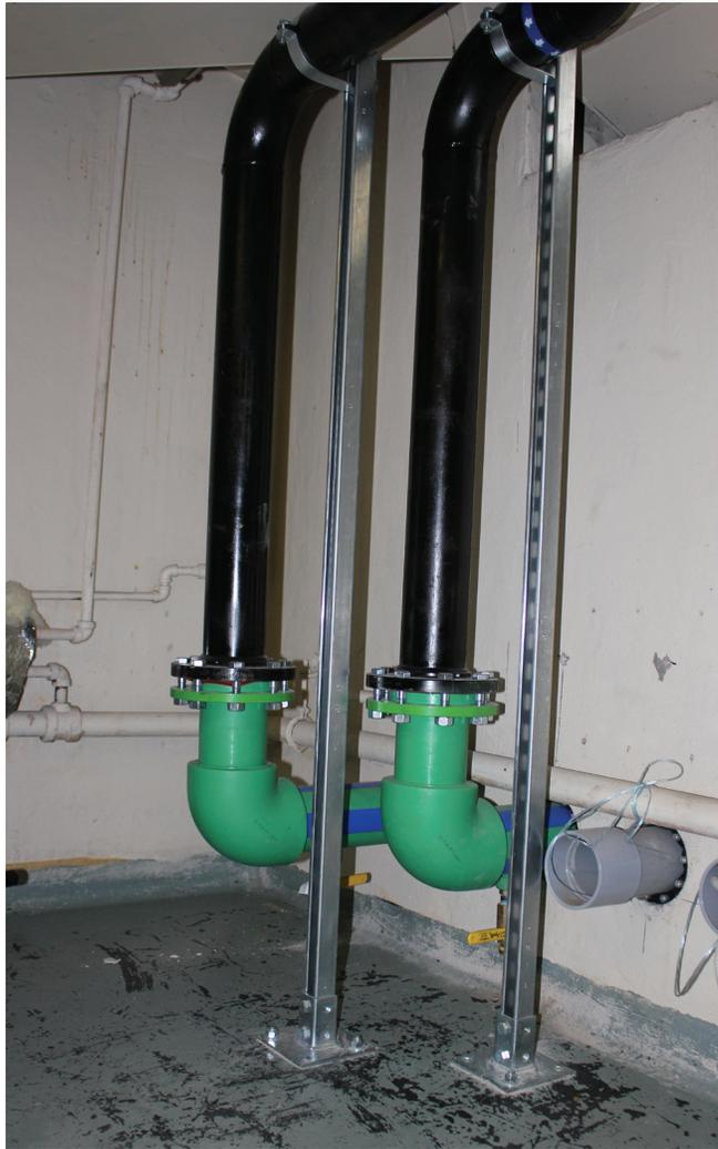
Using Aquatherm in lieu of steel also presented savings since the former didn't require insulation. "Since it's heat pump water, it's not too hot or too cold and the pipe has some insulating value so we didn't need to insulate it in the ground," Bobrowski explained.
