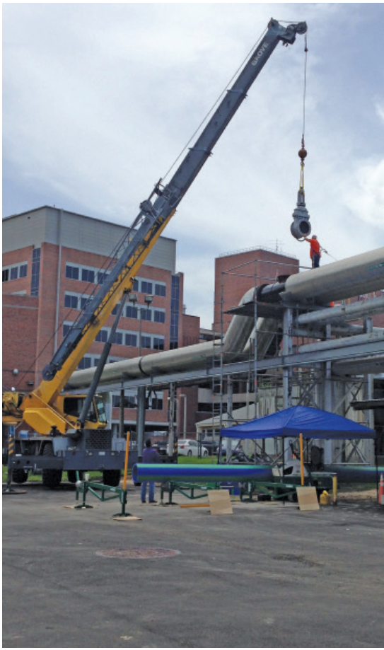
A crane lifts a 20-in. valve into place in an elevated section of the piping structure. Note the Aquatherm fabrication station under the tent in the bottom center.
