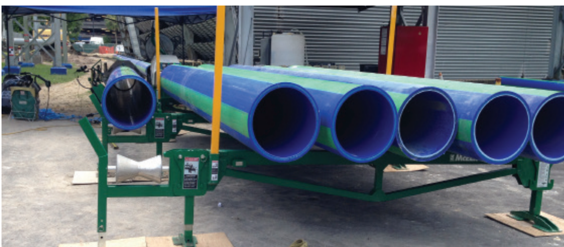
The McElroy PolyHorse pipe-handling system had the large-diameter pipe all loaded up and ready to be put into place for fusion connections.
