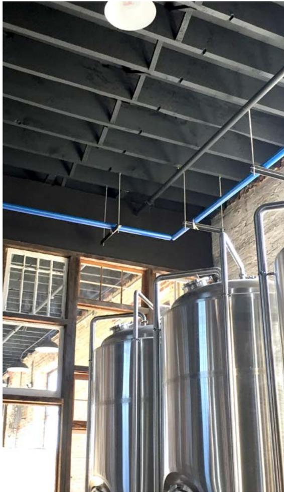
Fusion outlets are easy and can be installed very quickly. They can be added simply by drilling a hole into the existing pipe and heat-fusing a fitting directly to the pipe wall, so that there is no need to cut through the pipe and insert a “T” to accommodate additional branch piping. The system passed all leak tests and inspections without issue.
