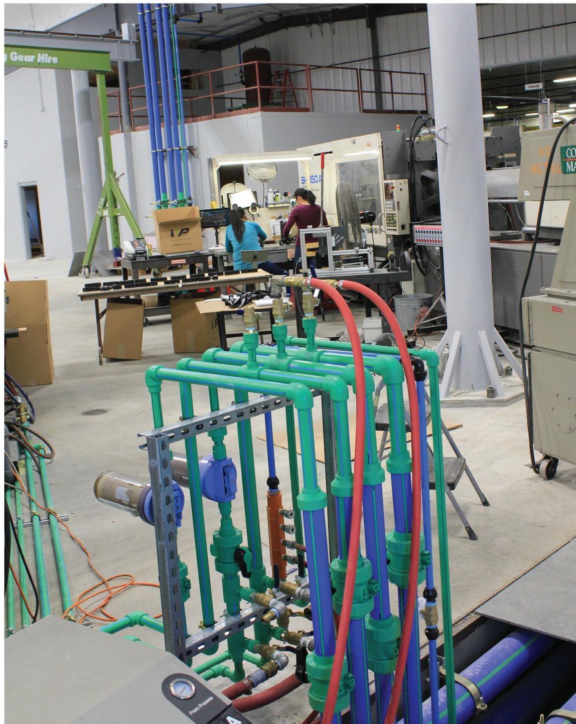
This project incorporated nearly 2,000 ft of Aquatherm Blue Pipe® for the process chiller piping, and 500 ft of Aquatherm Green Pipe®.
