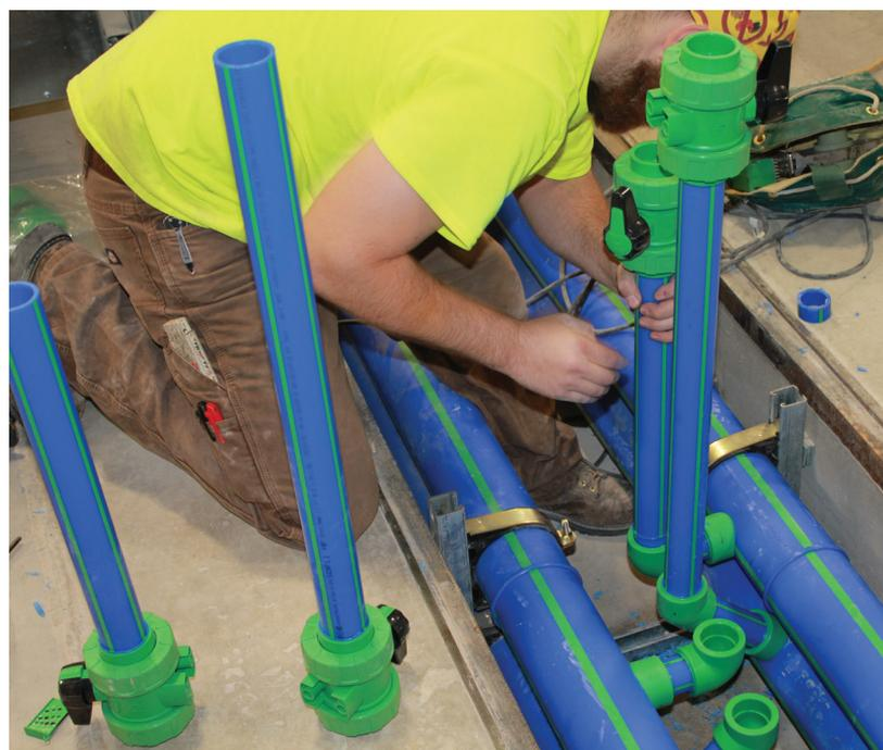
*Aquatherm pipe being installed at IVP Plastics. The plant's manufacturing machines may be moved into place and hooked up to the process cooling system as necessary.*
