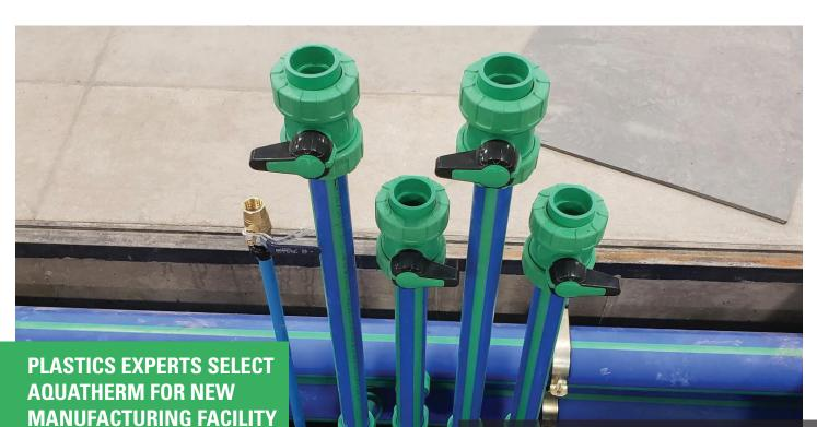
Aquatherm Blue Pipe<sup>®</sup> placed in a trench beneath the floor offers flexibility for this facility's process cooling needs.
